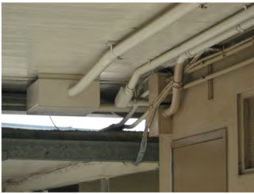
multiple buidling systems added/modified since original construction
