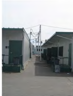
Interim classrooms during construction - 4 relocatable classrooms beyond to remain
