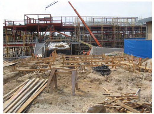
2-Story Classroom Bldg - from East
