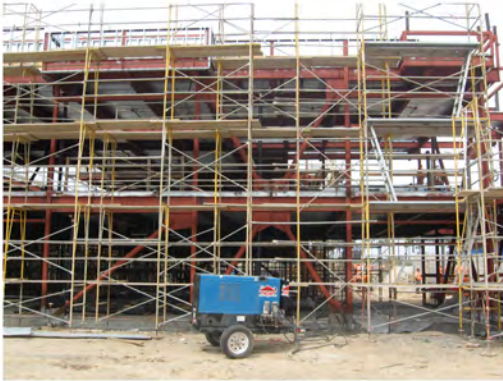
Note extensive cross bracing to meet earthquake standards very evident
