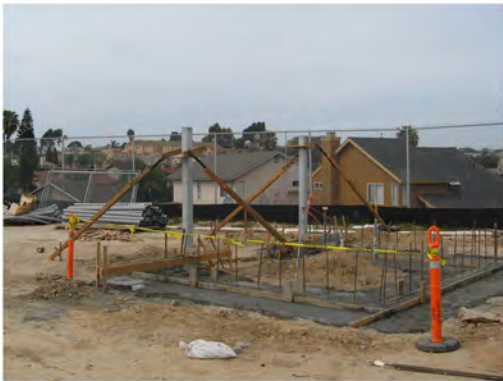
Foundation for new sewer pumping station w/ emergency power backup
