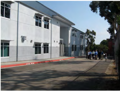
New 2-Story Classroom bldg
