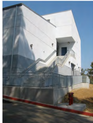
New 2-Story Classroom bldg
