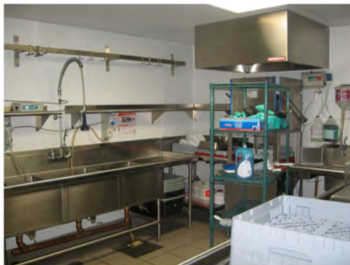
new scullery room
