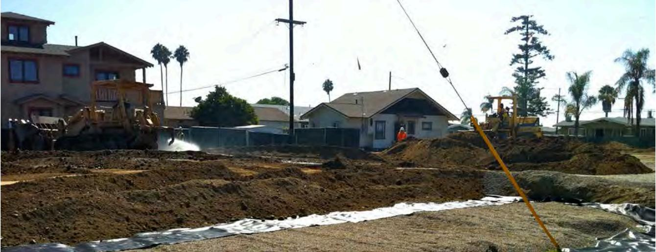
Earthwork underway for new artificial turf joint-use field (note: dust control measures seem to work well, no dust observed)
