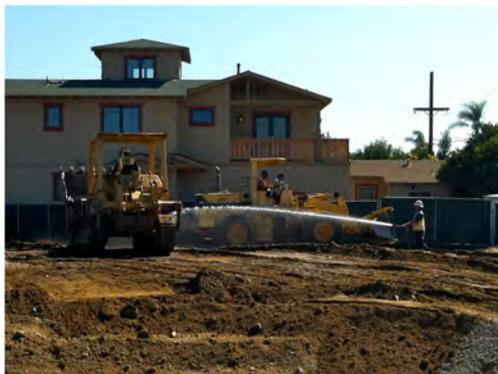
dust control during earthwork for new joint-use field (site expanded through street closure)
