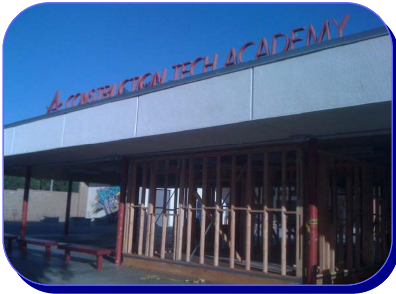
Kearny H.S. Construction Tech Academy First Prop. S Project
