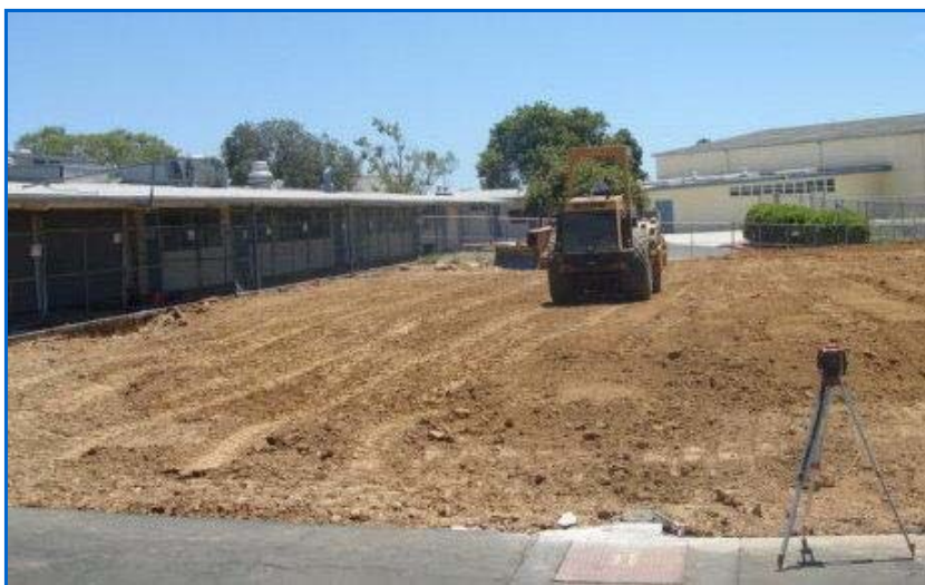
Construction begins on Clairemont High School's automotive facility.
