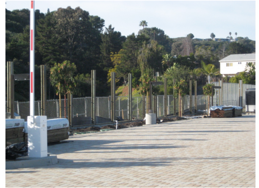
Landscaping & Sound wall along West side of campus
