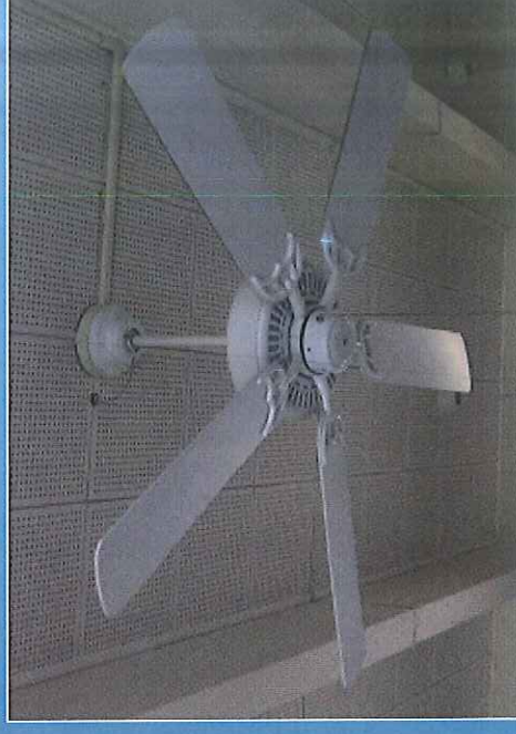
Ceiling fan installations at Sessions Elementary School
